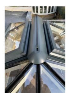
5. Fix the top cap to the base unit using the 40mm self-tapping screws provided. Make sure the cap it fixed tight down onto the base unit and is sitting square.
