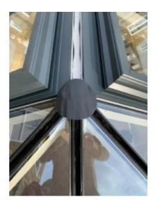
2. Then place the bottom section of the two-piece ride into place, evenly between each apex covering half the DPC disc and ensuring it is sits directly above the hexagonal timber block below the glass.
