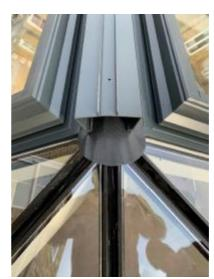
3. Fix the aluminium section in place with The screws provided. Ensure there is Even firm pressure between the gasket Running along the ridge cap and the double glazed units to provide a seal.
