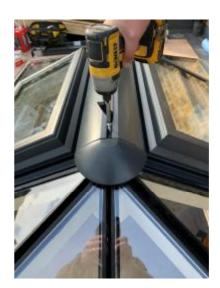
Now insert the black rudder gasket Making sure it is fitted tight up to Each cased end.
